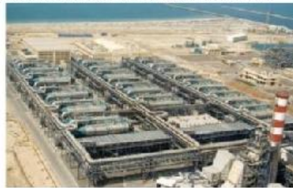
Gambar 32. Desalination Plant (Sumber: Utilities Middle East)
